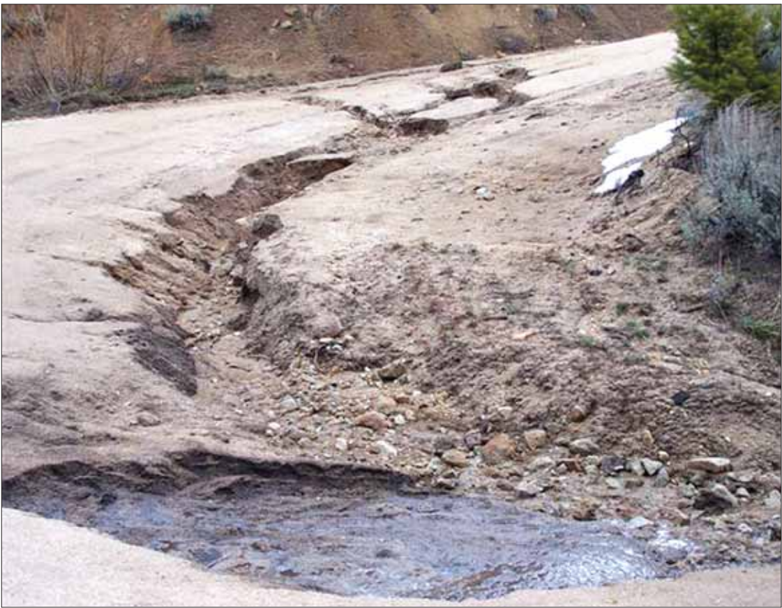
Scotch Bob Creek continues to flow over the Silver City Road last week, causing additional damage to the area already devastated by January flooding. High run-off is hitting the area as the area snowpack begins to melt. Mud slides also have struck the road, which is still in need of repairs from damage suffered in the original New Year's flooding. Photo by Larry McDaniel
